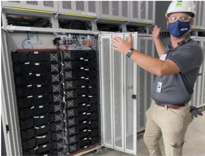
Vistra website photo, 22 battery modules in a rack
