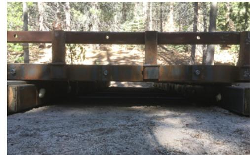
View of the underside of an elevated road segment constructed for the Yosemite toad/Cheryl Brehme, USGS Western Ecological Research Center
