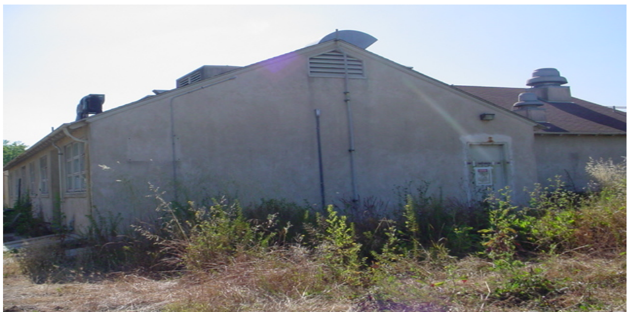
Figure 5-2, Hybridoma Center rear entrance showing ventilation exhaust systems and side view
