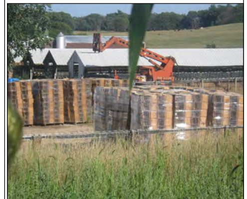
RENOVATION OR DECONSTRUCTION. GOLDEN SANDS RANCH WILD ROSE, WI
